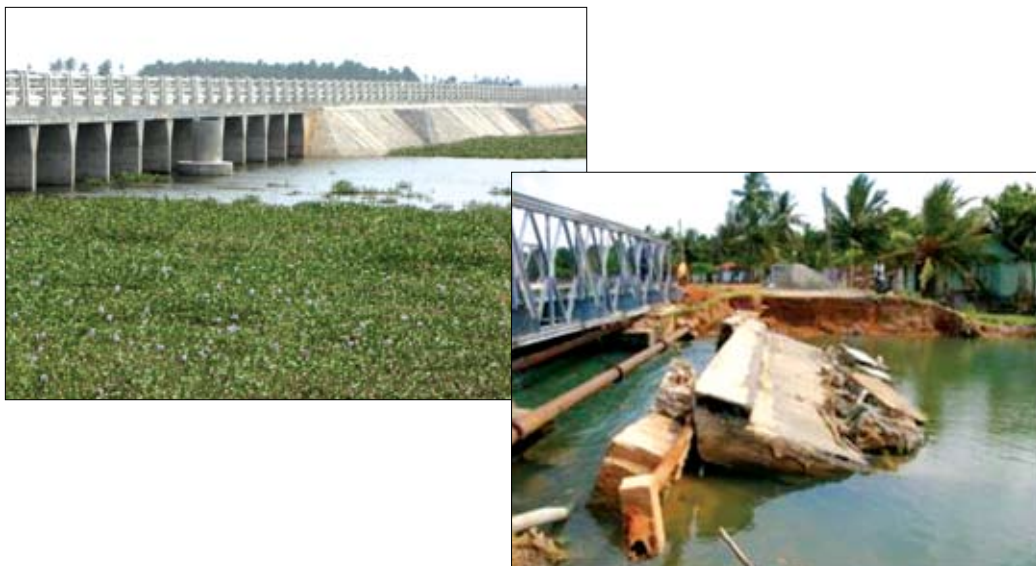
Figure 3.4 The new Periyakallar Bridge built with assistance from the Japanese International Development Cooperation Agency (JICA) has provided tremendous benefits through improved transportation, access to markets and trade. The adverse impact includes obstruction of water flow and acceleration of sedimentation. The reverberation effects of impeded drainage include water logging of paddy fields. (©J. I. Samarakoon)
