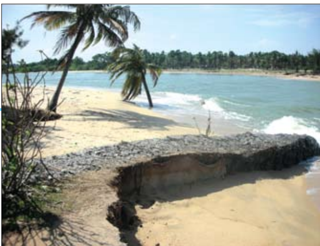
Figure 3.5 The road constructed by RDA with ADB support as a post-2004 Tsunami response had to be breached to ease the 2010/2011 flood. This road replaced a previous bridge that allowed drainage. (©J. I. Samarakoon)
