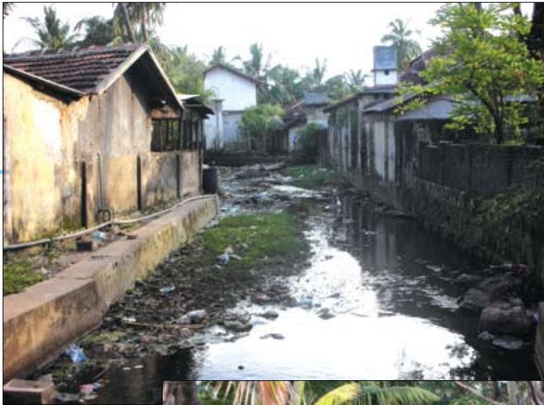
Figure 3.11 The drainage canal from the Batticaloa Lagoon (northern segment) to the west of Ertavur was designed to convey excess flood water to the sea. The paddy lands contiguous with this lagoon segment has expanded parallel with the supply of irrigation water from Maduru Oya development. Impeded drainage reportedly causes severe flood damage to life and property.
